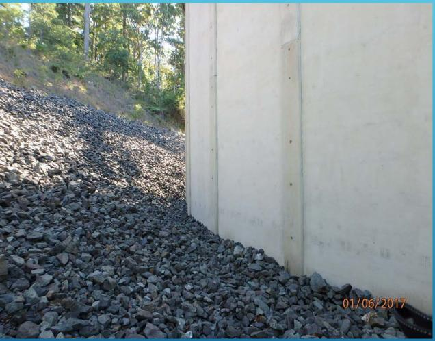
The backfilling has caused the walls on this tank to spall in the middle areas, after three years in service.
