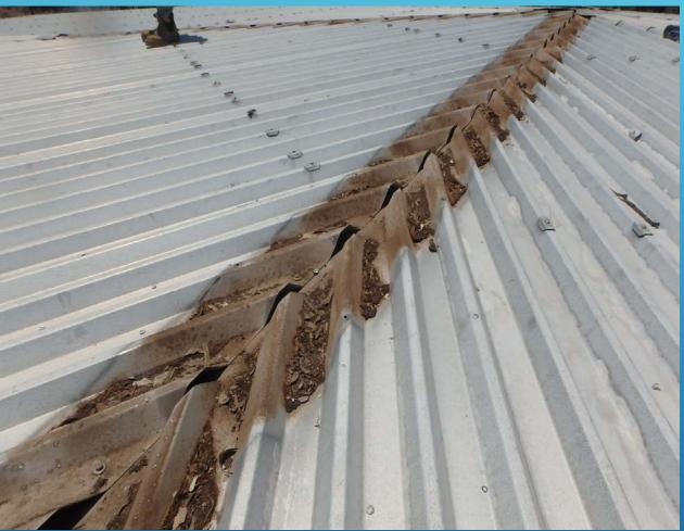
**Number 3:** Placing safety mesh under the roof sheets to comply with OH&S during construction. This material is usually the cheapest available and corrodes quickly, causing the roof sheets to fail and then dropping the debris down into the tank and making regular cleaning of the floor difficult. In a factory situation, there would have been a layer of insulation between the mesh and the roof sheets.
