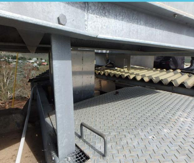
Entry hatches mounted too far off the wall, so that ladder supports have to be extended to accommodate the excessive distance.
