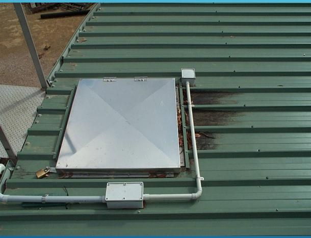
Flashings on the edge of roof areas prevent rain water from draining off and ridge cap flashings are difficult to seal and allow all sorts of debris, bird nesting and vermin entry to occur.
