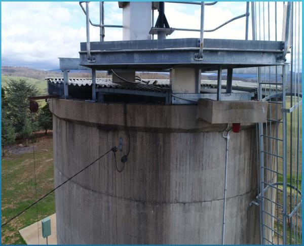
The entry hatch cover was then made up as an extended section and dropped down into the open roof hole. It wasn't sealed onto the new platform area around the edges, but below the platform was a far worse sealing issue!
