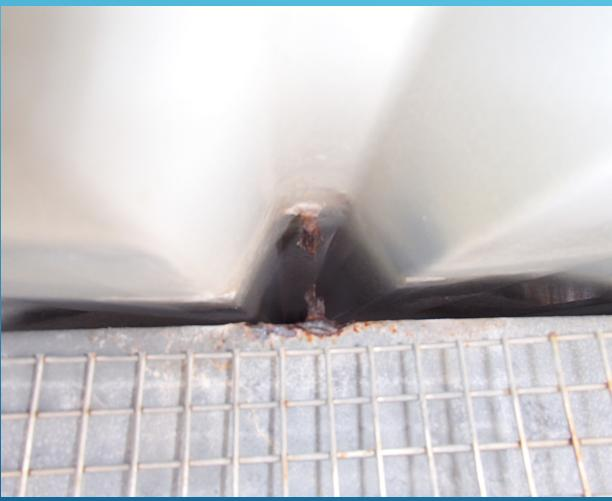
**Number 6:** Platform and entry hatch designs that limit working space and safe access into and out of the tank. What may be suitable for a factory environment is different to an elevated, confined space application, where diving and rescue equipment is commonly used. Platforms mounted high over the entry hatch area, instead of being level with the roof.
