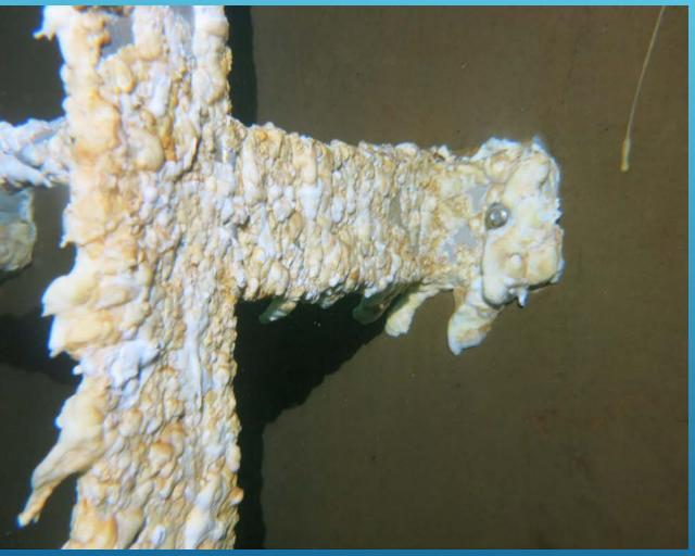
**Number 9:** Not thinking about how internal pipework will affect the stored water quality. Inlets placed next to outlets lead to short circuiting issues. Outlets close to the floor allow sediments to be drawn into the downstream reticulation system. Scours not being fitted in the lowest area of floor will not allow for effective draining of the tank.
