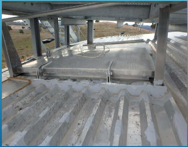
The worst platform outcome identified to date! A new platform was constructed over the top of the existing one, which was partially removed, leaving a large unsealed area leading directly into the tank.
