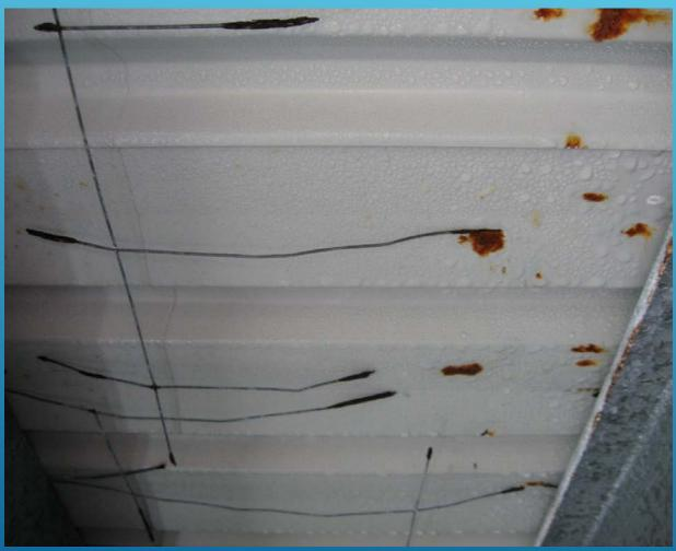
The corroded safety mesh breaks away and drops down onto the floor area, making effective tank cleaning a near impossible task. It also corrodes the roof sheets from the underside, leading to structural failure and an unsealed roof surface.
