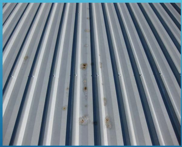
**Number 4:** Using roof framing materials that are not suitable for hot, moist and gaseous conditions. Zincalume coated purlins and rafters have a short life span in these situations and they also deteriorate quickly when roof screws puncture the surface coating.
