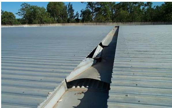
Figure 5 Collapsed roof gutter
