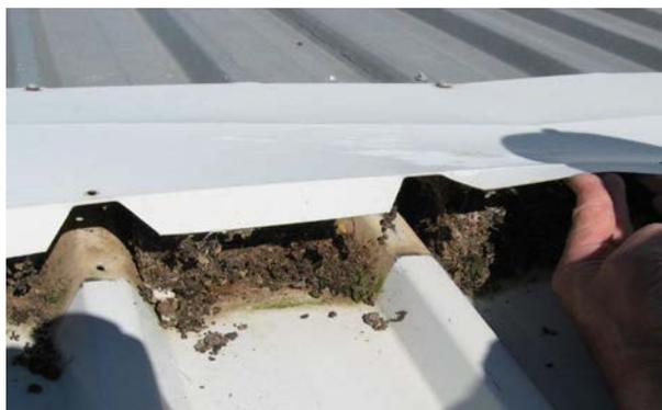
Figure 6 Debris build-up under roof flashing
