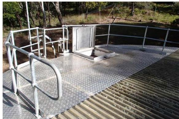
Figure 4 Good platform and hatch design
