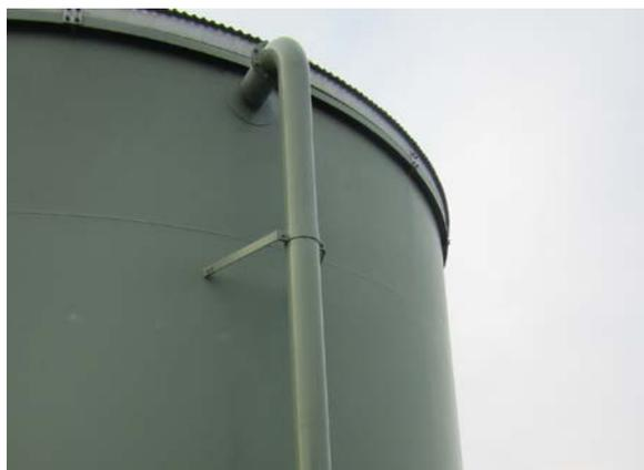
Figure 7 Through the wall, external overflow
