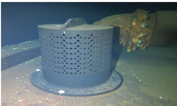
Figure 10 HDPE outlet screen – close fitted, good result
