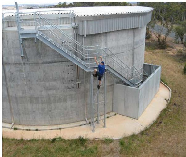
Figure 2 Security measures easily by-passed
