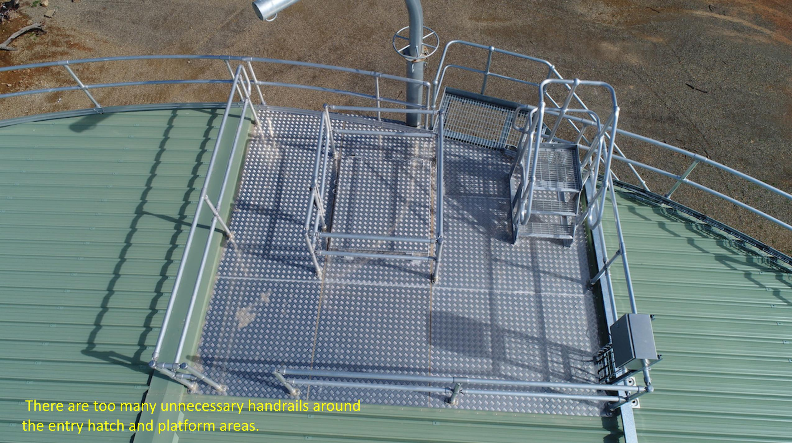
There are too many unnecessary handrails around the entry hatch and platform areas.
