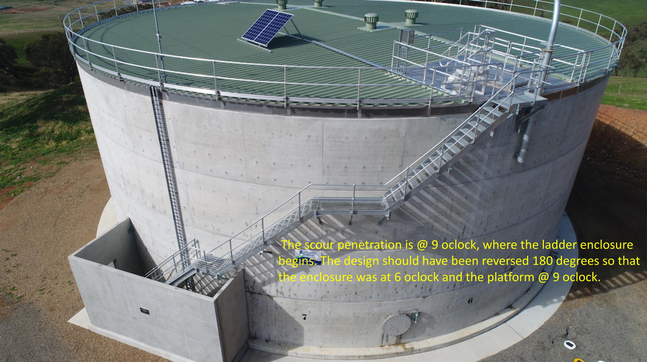
The scour penetration is @ 9 oclock, where the ladder enclosure begins. The design should have been reversed 180 degrees so that the enclosure was at 6 oclock and the platform @ 9 oclock.
