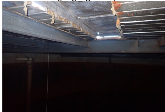
Sever corrosion on roof members or sub-standard light gauge components
