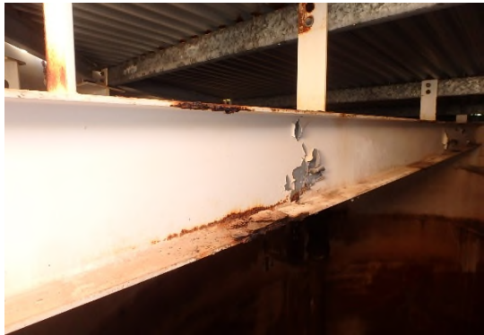
Sever corrosion on roof members or sub-standard light gauge components
