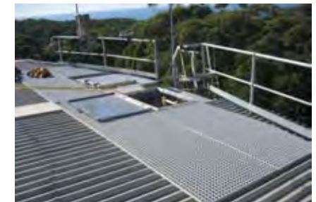
After platform renovation
