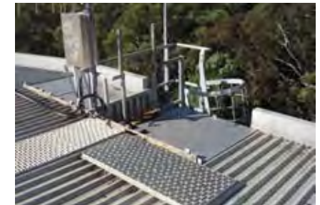
Before platform renovation
