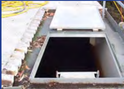
Entry hatch after
