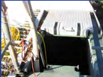
Entry hatch before
