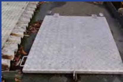
New entry hatch closed
