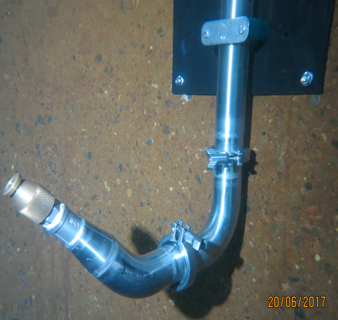
Aquajetta nozzle fitted inside a concrete tank
