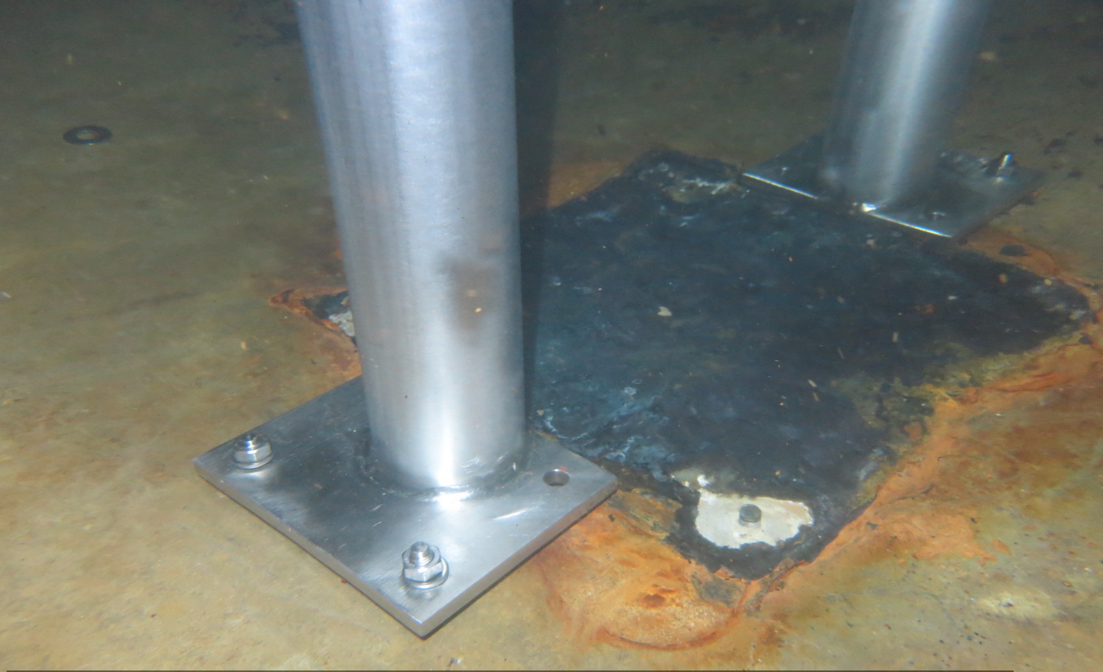
The base section fits around the existing post, which is then removed
