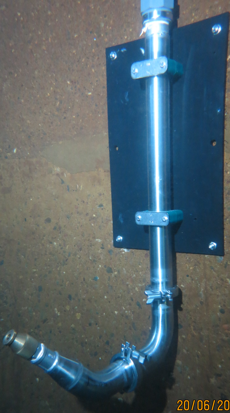
Aquajetta nozzle fitted inside a concrete tank
