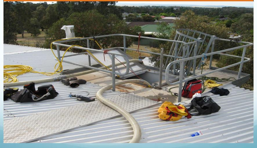
The under side area of the platform – this simple plumbing job was carried out using 'off the shelf fittings' while standing on the internal ladder
