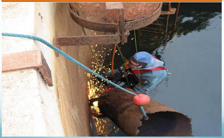
The support brackets on this overflow riser pipe are galvanized and beginning to corrode, while the epoxy coated areas are still OK.
