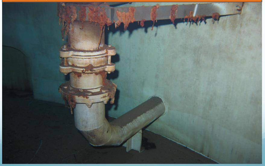
This roof support post was galvanized instead of being epoxy coated like the wall and floor areas of the tank.
