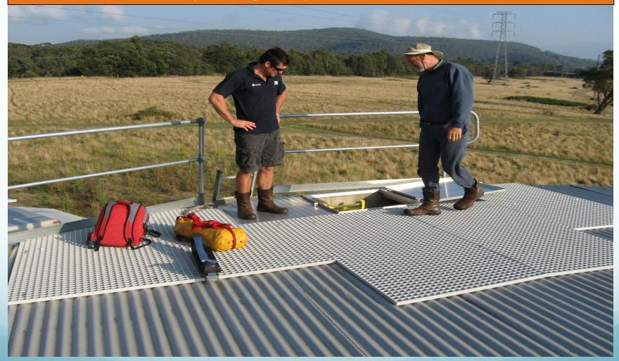
Another simple renovation – extra guard rails, a new overlapping hatch cover and the adjacent roof sheets protected to increase the available working area.
