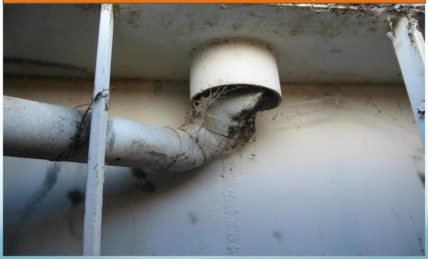
Another example of a roof drain which is not connected into anything – this was very simple to fix once it was identified.
