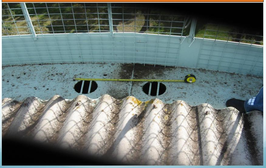
A piece of 90mm storm water pipe is simply pushed inside a 150mm drain point – and expected to prevent excess water and contamination from entering the tank!
