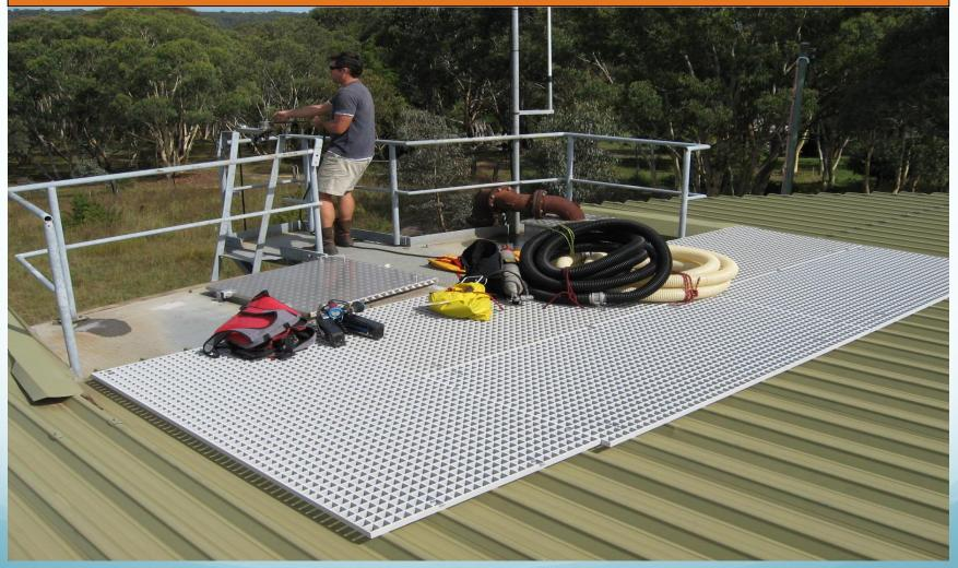
A new enlarged and fully sealed entry hatch, additional guard rails and an 'open plan' working area – note the telemetry control box located in a sensible position.
