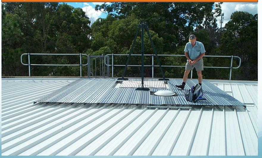
This is a concept design for a good platform area – open plan, plenty of working space and a rescue system in place to suit confined space requirements.
