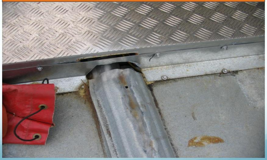
Another close up of the new platform area and how the roof now drains directly into the tank. Good design would have overcome these issues and made the project worthwhile.
