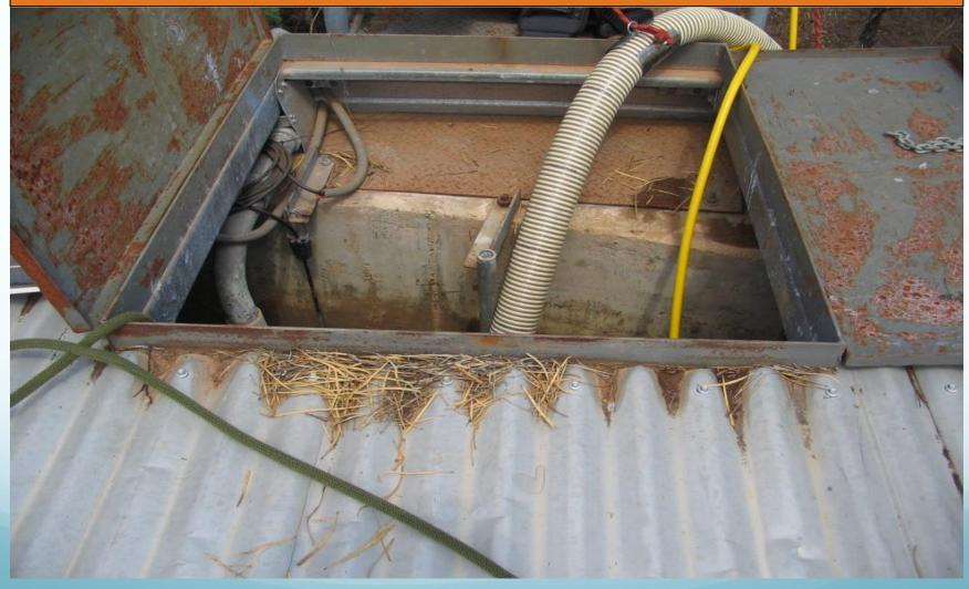
A significant hole has been cut into the platform area to service a sensor unit – all this accumulated material is finding its way into the tank.
