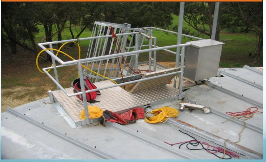
A close up of the platform to roof sheet sealing and a lack of understanding regarding the upgrade process and what it was supposed to achieve.
