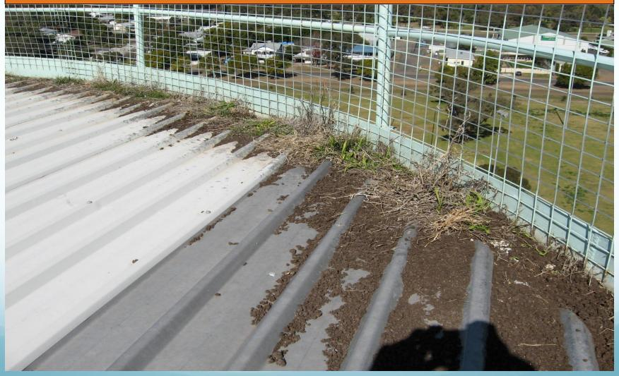
The roof sheets are fastened directly onto the hatch frame and have no means of draining water and debris away from this area - the ponded water leaks into the tank.
