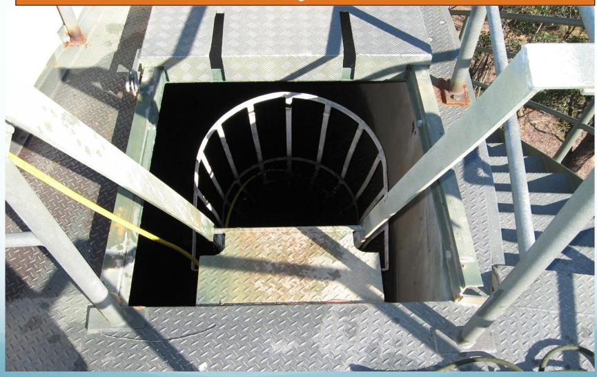
The ladder stiles extend out through the opening and the hatch cover is not sealed or secured
