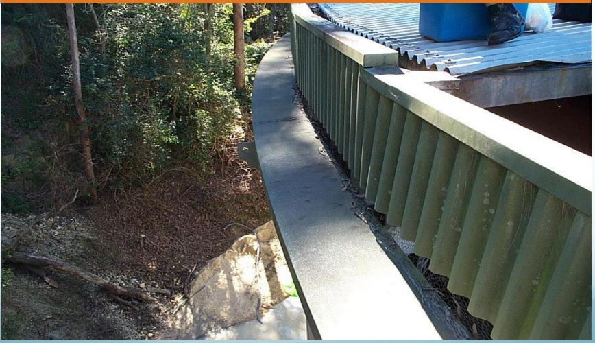
This ventilation is poorly designed – the mesh is too coarse and not sealed along the lower edge, where contamination and debris is collecting and entering the tank.
