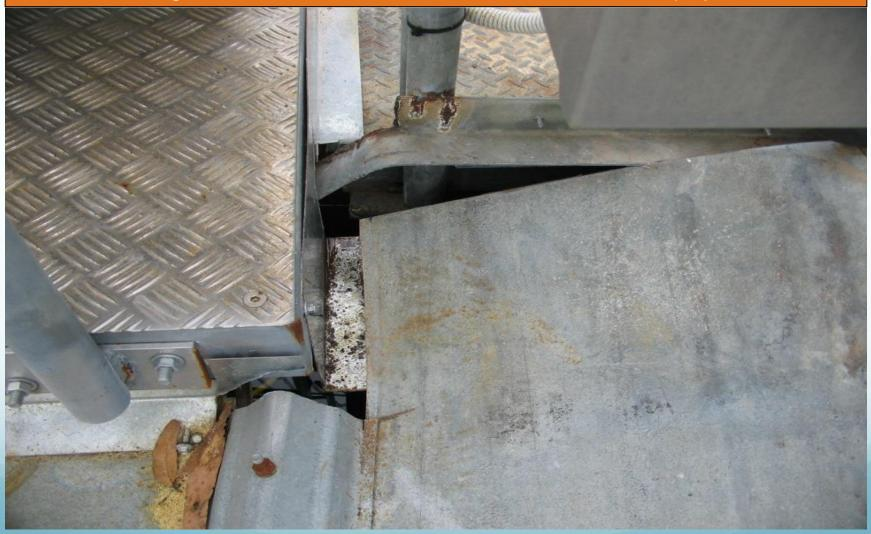
A new roof and platform, however a roof vent was placed right in the middle of the working area – this DOES count as a trip hazard!
