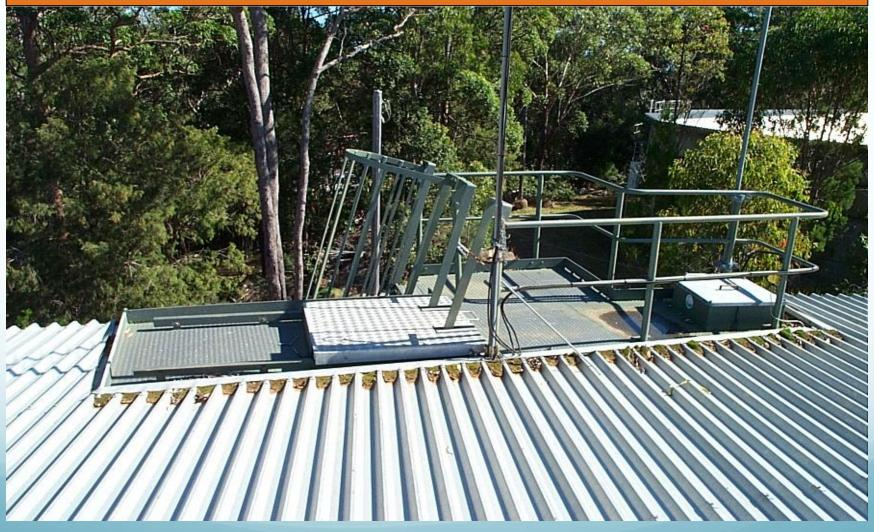
The working space is too small, the entry hatch is unsealed and the whole area is covered in bird faeces and debris. The adjacent trig tower is encouraging birds to roost in this particular area.
