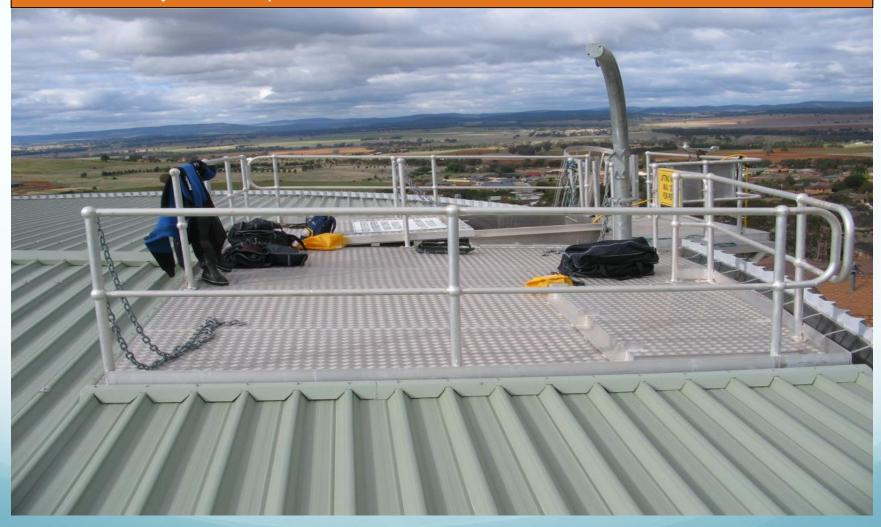
A simple 'open plan' upgrade on a small tank – adequate guard rails around the sealed hatch area and FRP mesh protecting the adjacent roof sheets.
