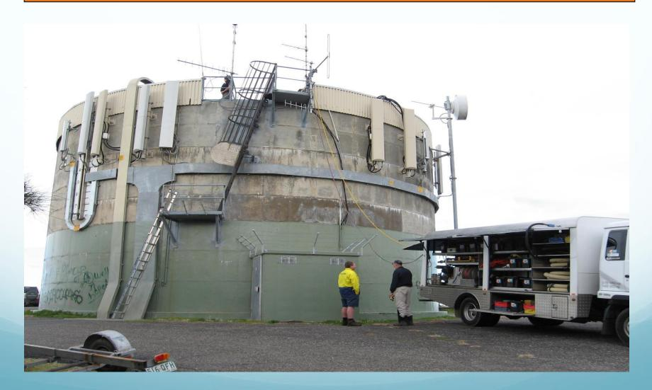
This platform requires guard rails on the LHS and the entry hatch area is unsealed. The adjacent roof sheets are ponded with debris and cannot drain away effectively .
