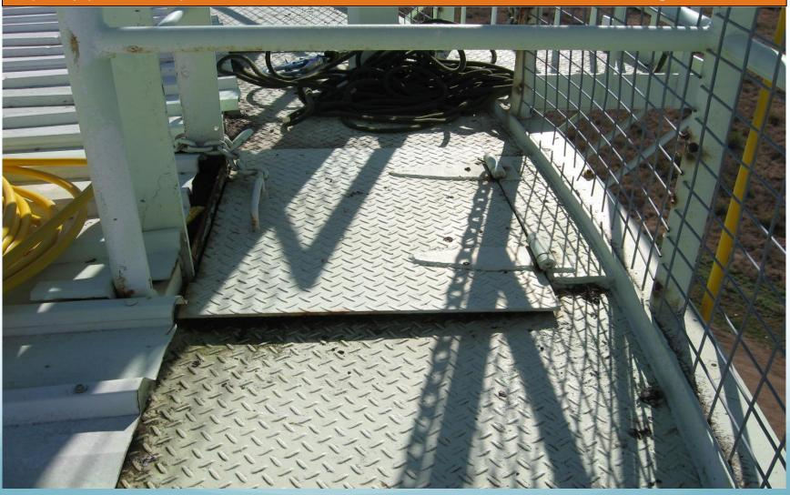
This entry hatch is too small for a confined space entry and it is poorly positioned on the platform. It should be parallel to and close to the wall area to allow for a more ergonomic placement of the ladder.
