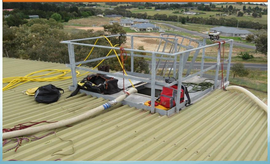
A platform upgrade with poor outcomes – personnel are 'fenced into' a small working area and the roof sheets are not sealed where the platform module was cut in.
