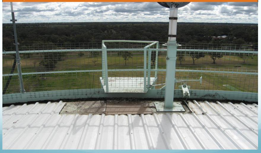
The working area is overcrowded with control boxes and other accessories, that could have been located further away to make room around the immediate access area.
