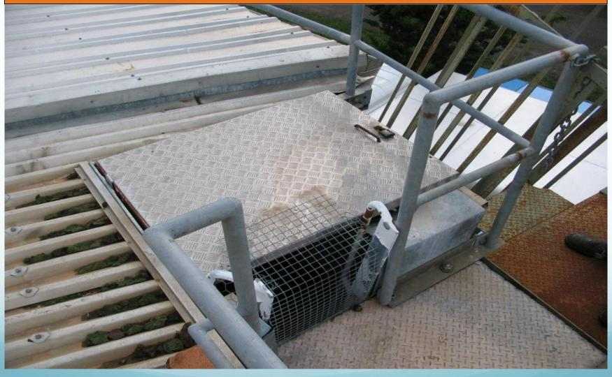
The entry hatch is too small for safe confined space entry and there is no sealing capacity present to prevent natural or deliberate contamination from entering the tank.
