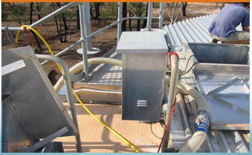
Personnel are 'fenced into' a small working section and have to continually climb over the rails to access the roof area - more guard rails are required on either side of the roof.
