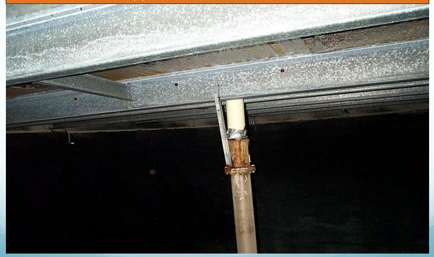
This box gutter has corroded away and is now draining all of the roof directly into the tank
