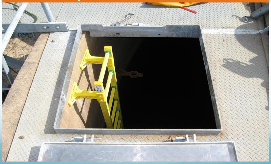
Entry hatches were mostly designed to keep out unauthorised personnel or larger vermin and rescue scenarios were not considered. The openings are often too small and the front edges of the hatch frame have been assessed as being a potential trip hazard to maintenance personnel - these raised edges were removed in most cases.
