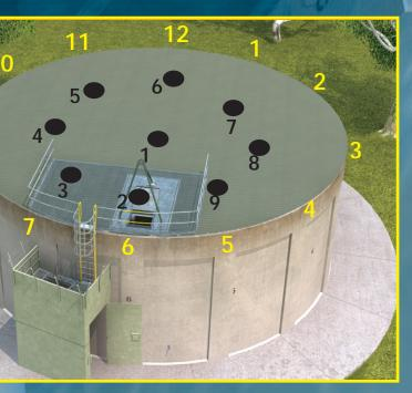
THE CENTRE POST IS #1 AND FURTHER NUMBERS RADIATE OUTWARDS IN A CLOCKWISE DIRECTION WITH #2 BEING NEAREST TO THE 6 O'CLOCK POSITION.
