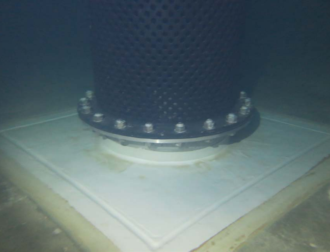
A flanged and sealed outlet base with an HDPE safety screen fitted
