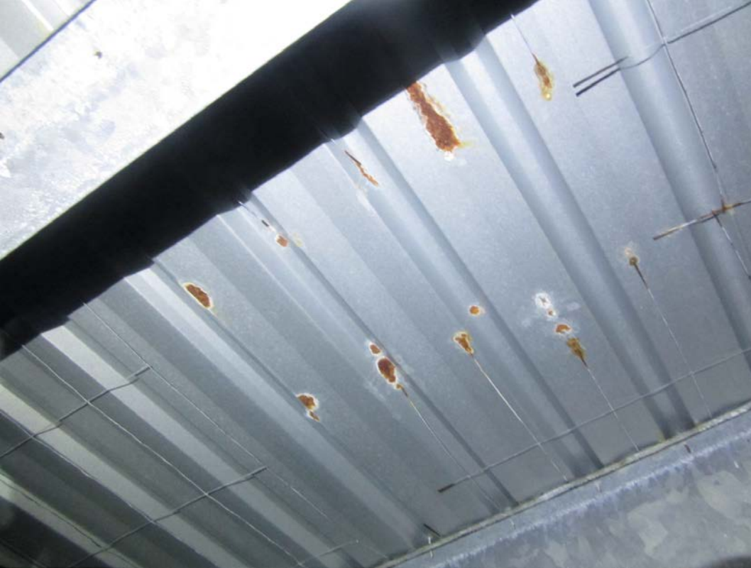
Roof safety mesh corroded and damaged sheeting
